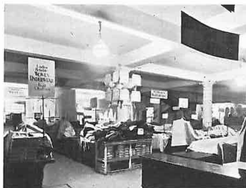
"HALF-WATT" LAMPS AT SELFRIDGE'S. A corner of the Bargain Basement lighted by Mazda "Half-Watt" lamps in Alba spheres. Where goods are sold below cost it is essential that the lighting should cost as little as possible. See?
